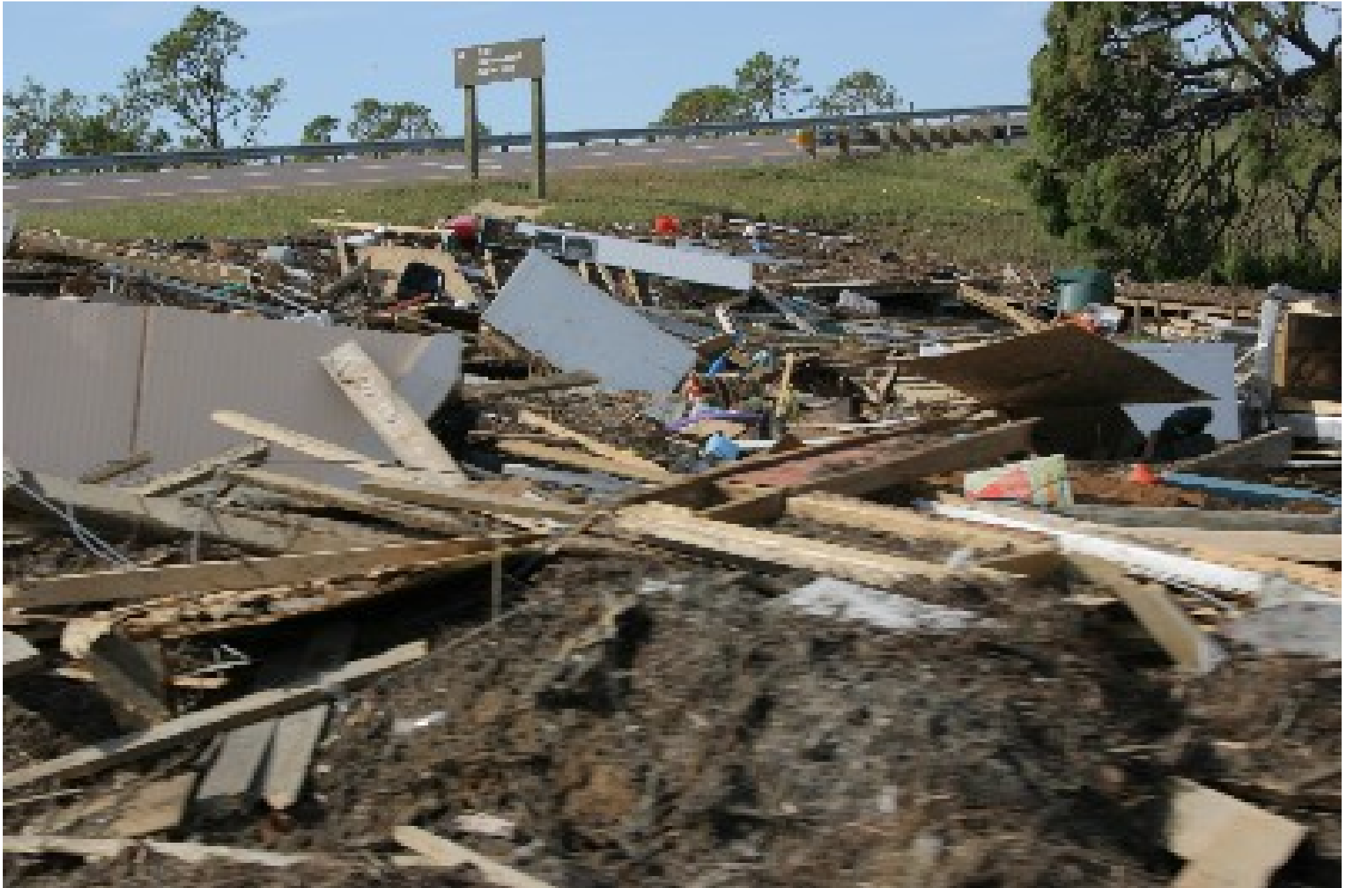
Debris field from Ivan storm surge, Perdido Key, 9/21/04.
