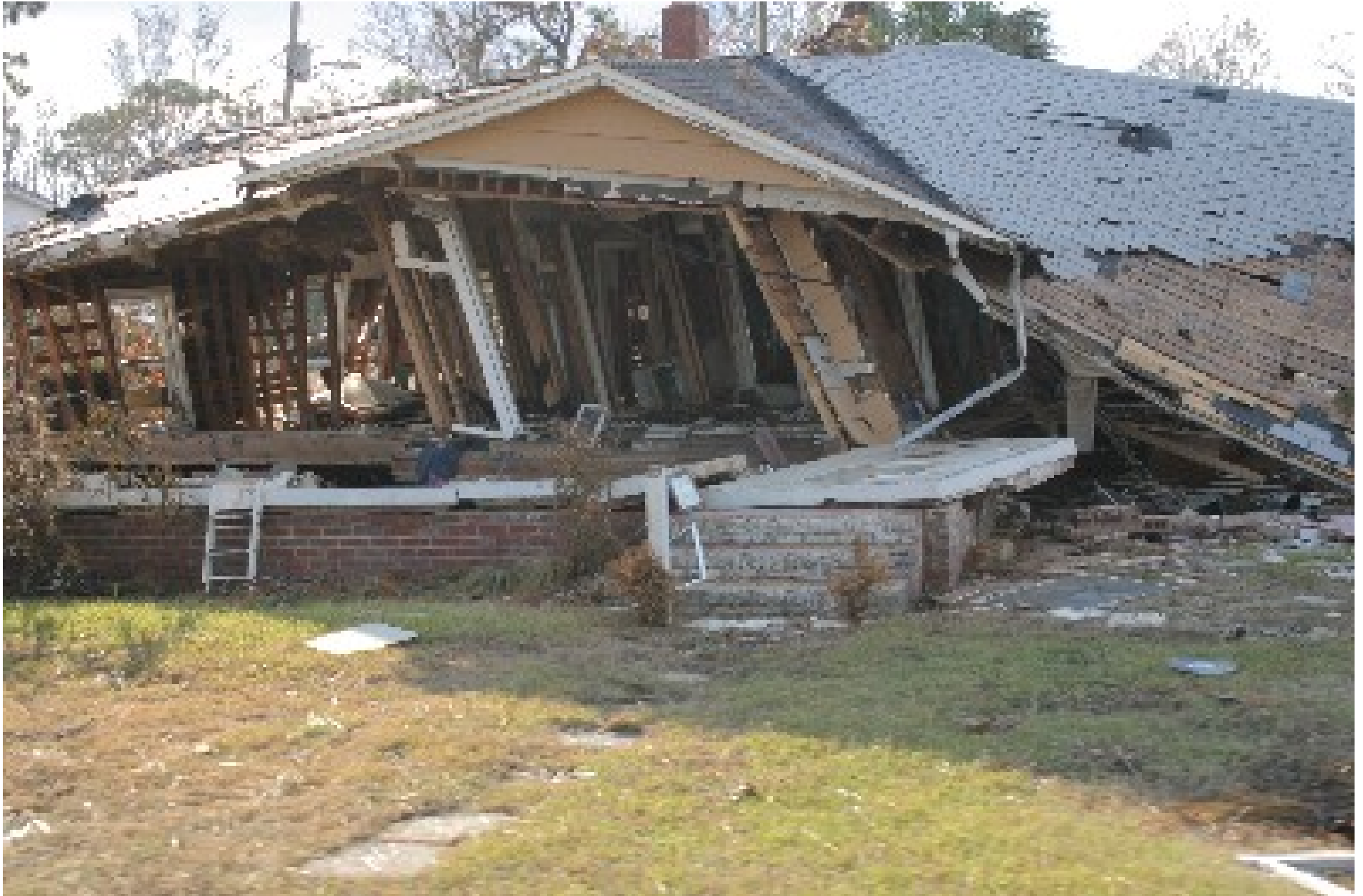
Home destroyed by Ivan, St. John the Evangelist parish neighborhood. 9/25/04
